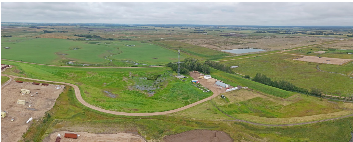
An aerial view looking west towards the Greenlight Electricity Centre site.
